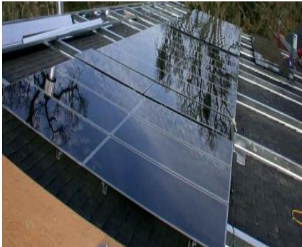
Frameless Thin Film Modules applied to roof top
